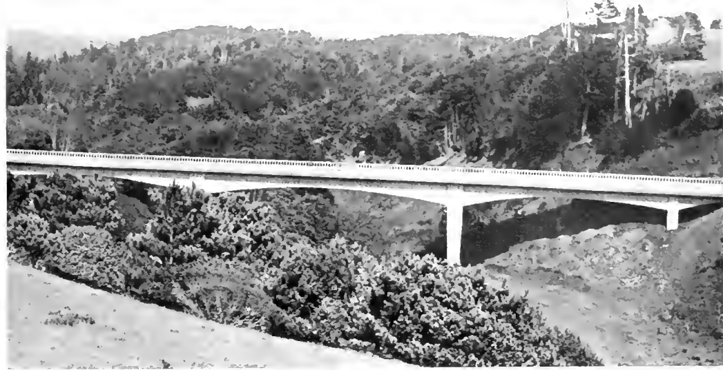
Side view of Schooner Gulch bridge shows simplicity of design
